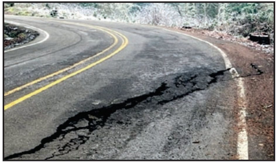
Above In North Douglas county out on Smithville Rd. Freezing water has played havoc on this county road. Asphalt is cracked open. Photos by Russ and Charlotte
